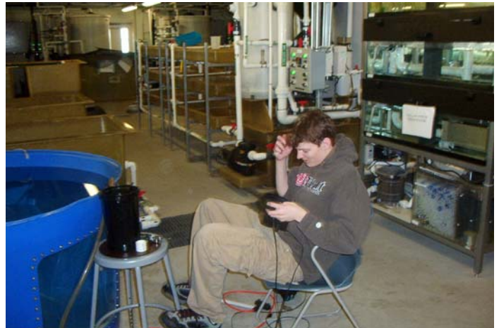
Pat figuring out the pump system needed
