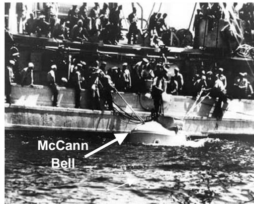
At the time of the Squalus incident, undersea rescue below the depth that a diver could operate was unthinkable. Momsen, however, had been working on an old concept of using a tethered diving bell (which dated back to the time of Aristotle) to attach to the rescue hatch of submarines, enabling the trapped seamen to escape and be hauled up to the surface.
